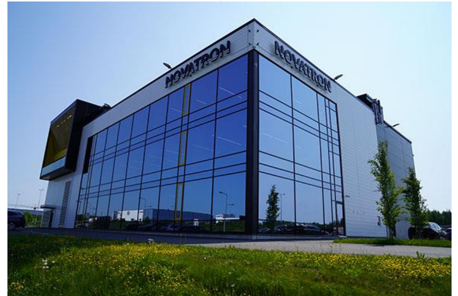
Technology Center in Pirkkala, Finland
